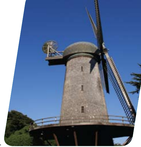
This Dutch style windmill in Golden Gate Park in San Francisco was built in the early 1900's to pump water from an underground aquifer to irrigate the park.
